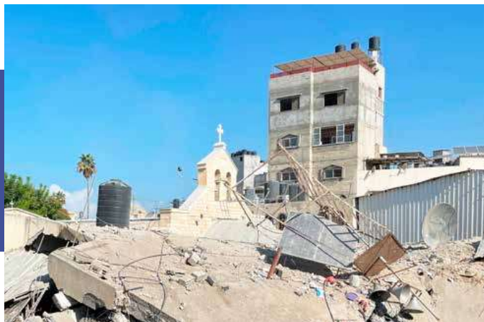
Remaining structure of a church among structural damage from air strikes.
