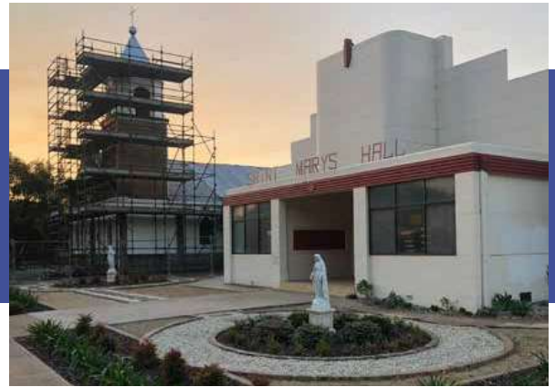
Above: Scaffolding is placed around the steeple.
