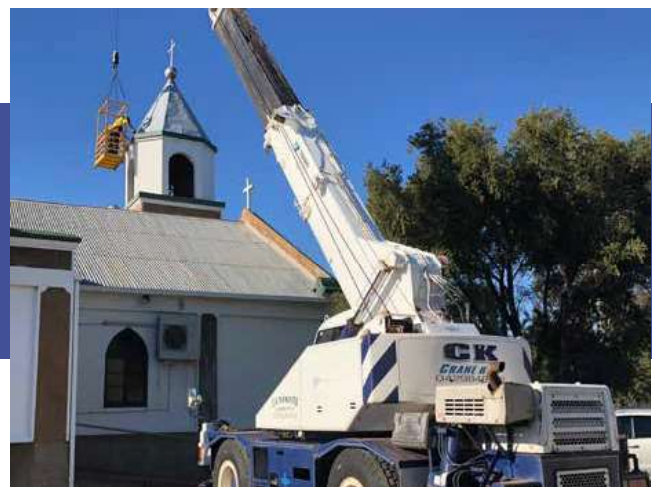
Below: A crane was needed to get to the steeple.
