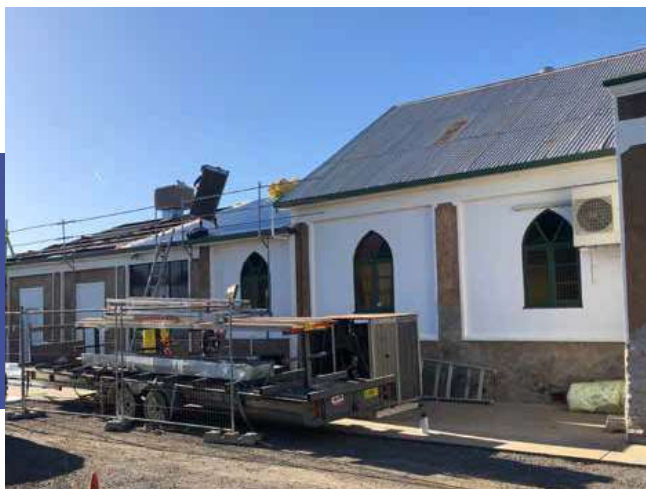
Above: Restoring the roof.
